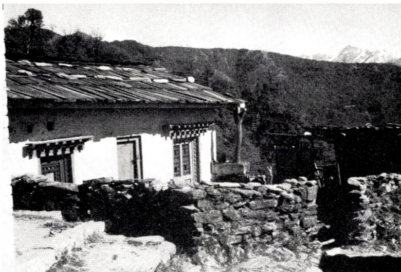
Fig. 16. A typical monk-house in Som-den-tho-ling. Stones are placed on the roof in order to hold it down in storms. In the distance, snow-covered peaks near the Tibetan border.
